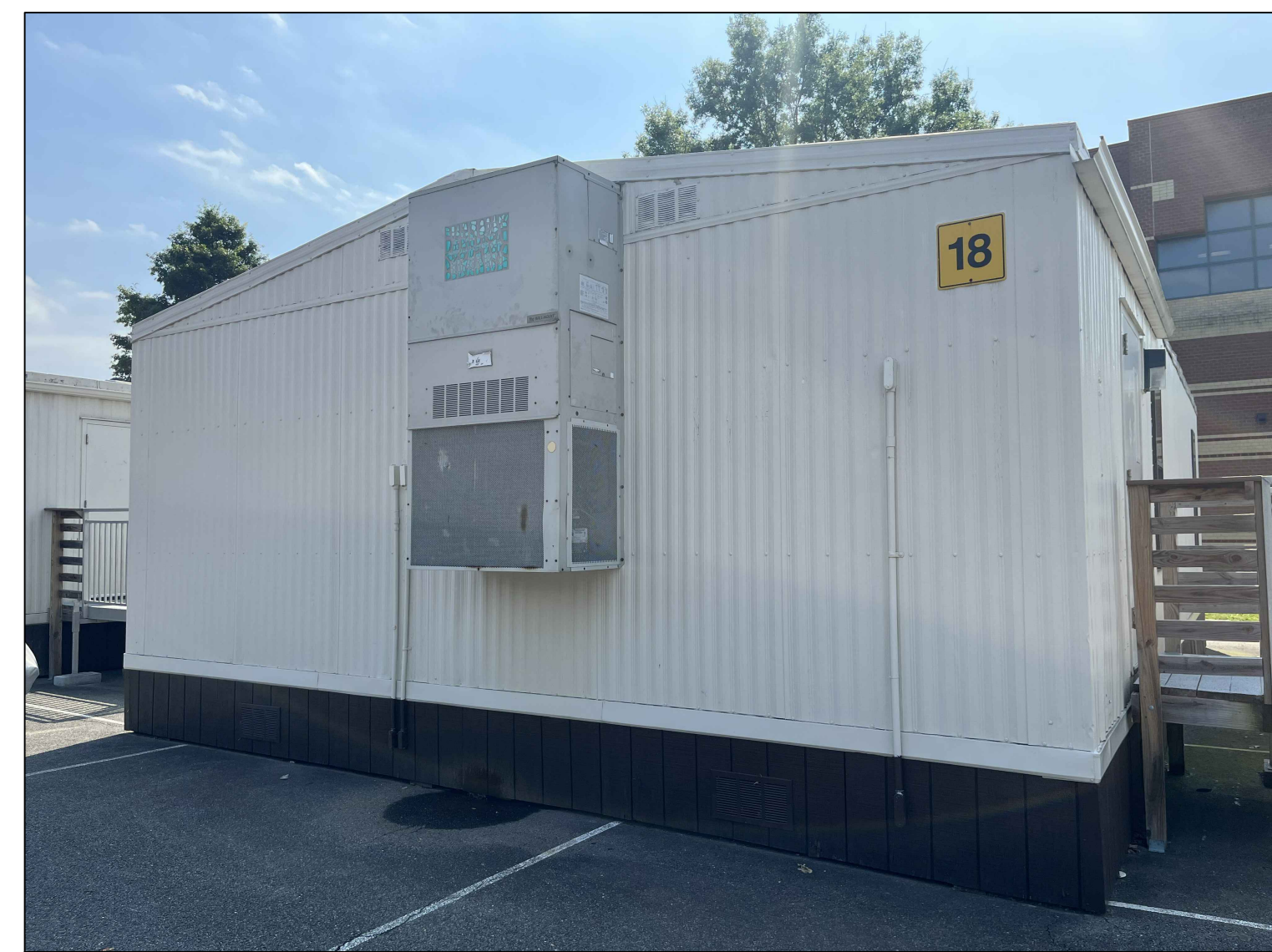
2 RESERVOIR HS RELOCATABLE CLASSROOM #18-EXISTING CONDITION PHOTO ME8.4 SCALE: NO SCALE
