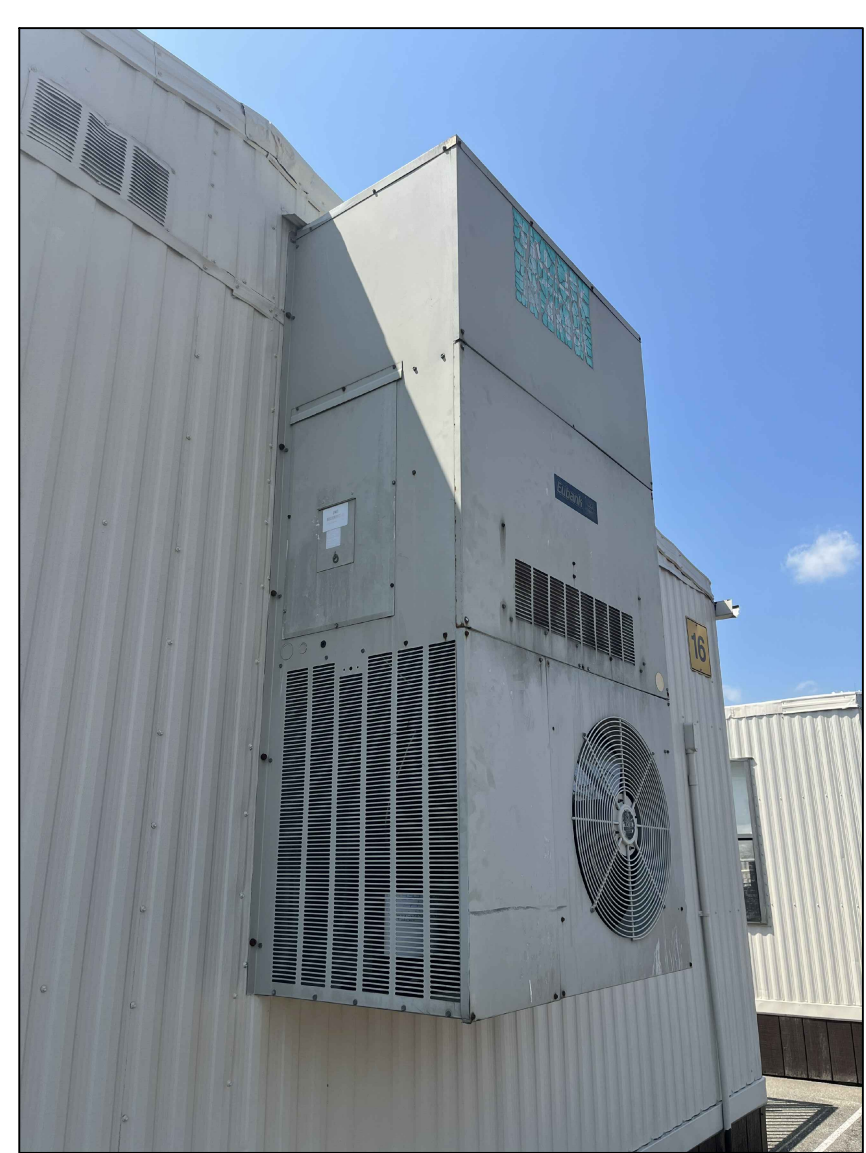
2 RESERVOIR HS RELOCATABLE CLASSROOM #16-EXISTING CONDITION PHOTO ME8.2 SCALE: NO SCALE
