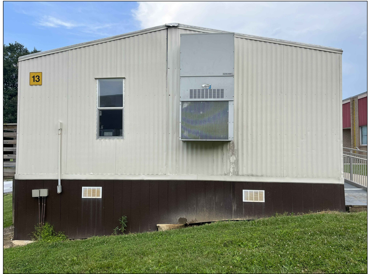
2 HAMMOND ES RELOCATABLE CLASSROOM #13-EXISTING CONDITION PHOTO ME4.2 SCALE: NO SCALE
