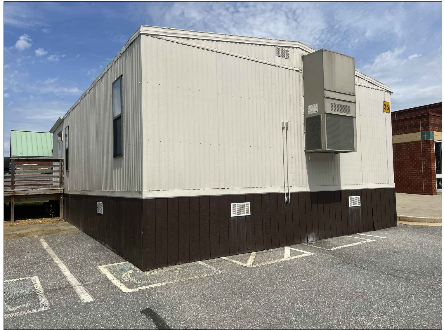
2 ILCHESTER ES RELOCATABLE CLASSROOM #35-EXISTING CONDITION PHOTO ME5.2 SCALE: NO SCALE
