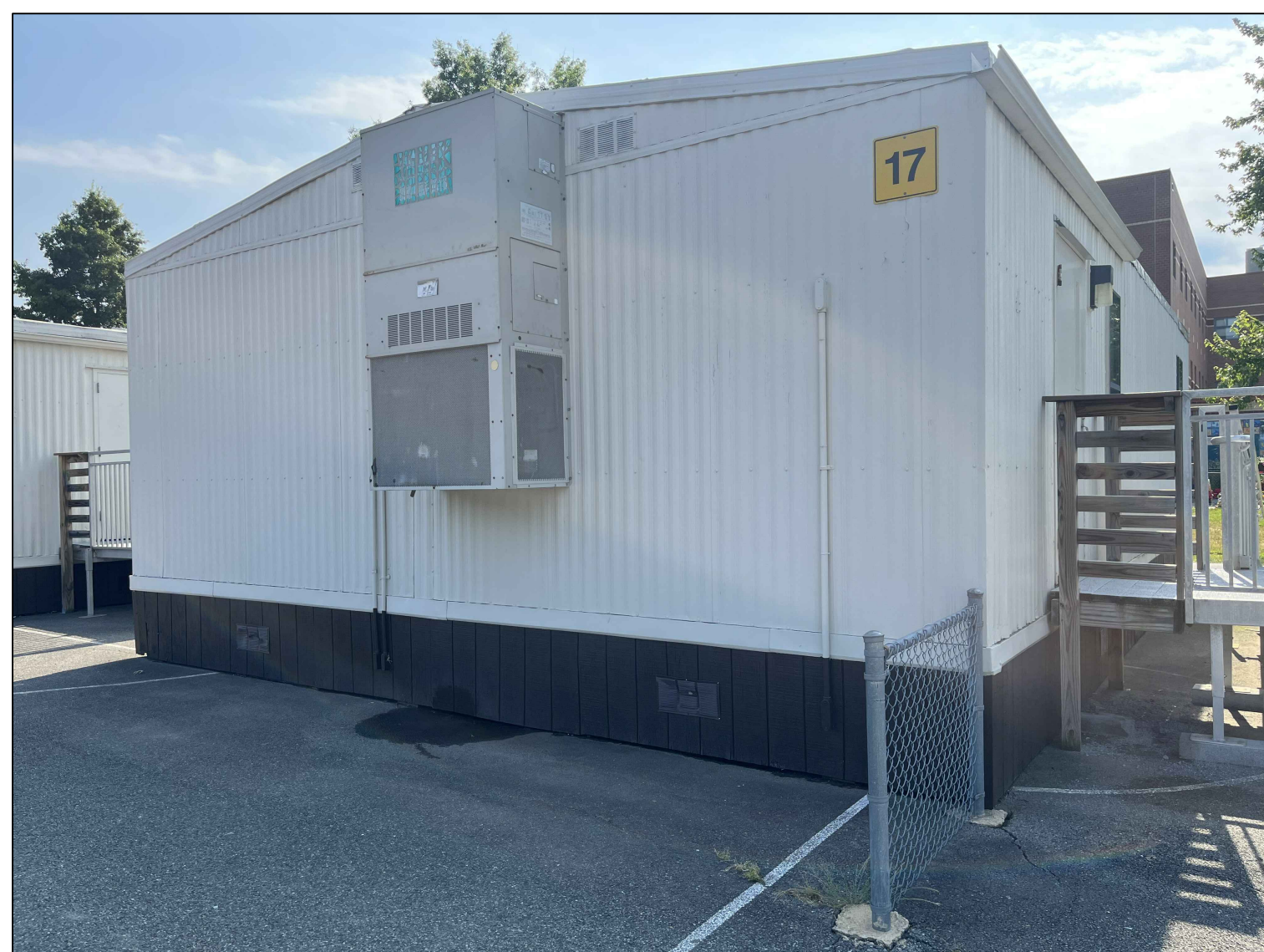
2 RESERVOIR HS RELOCATABLE CLASSROOM #17-EXISTING CONDITION PHOTO ME8.3 SCALE: NO SCALE
